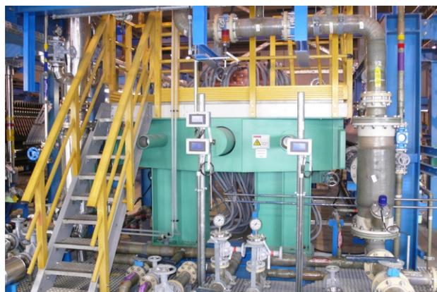
The mechanical and electrical equipment of the production plant is made of high quality, durable and economically efficient products. High quality materials with an outstanding corrosion protection (this includes special plastics, stainless steel and titanium) are used according to the requirements of the different media.
