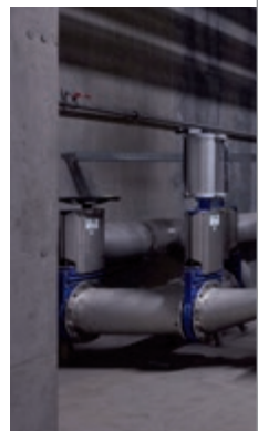
Inlet pipe secondary treatment
